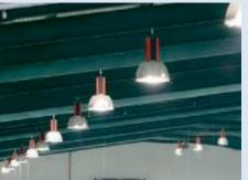
Double fluorescent with cheap reflector Suspended HP sodium Suspended HID Typical illuminance 500 lux
