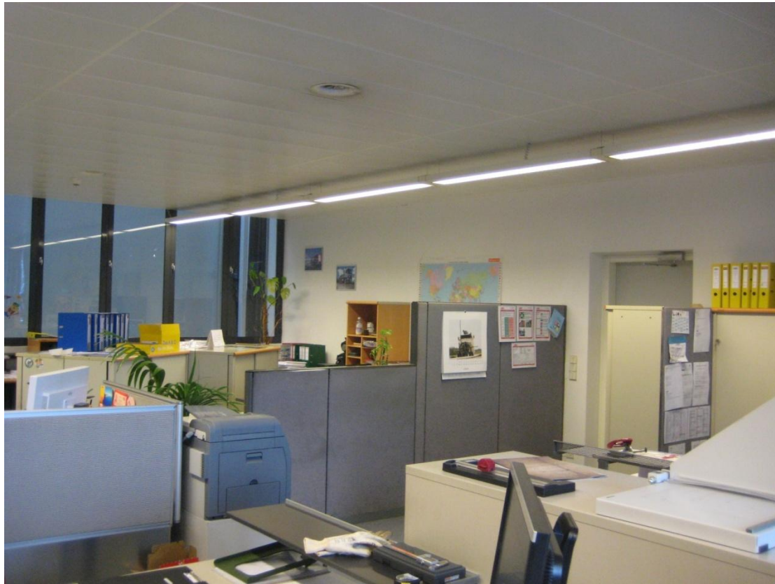
existing lighting (T8 technique)
