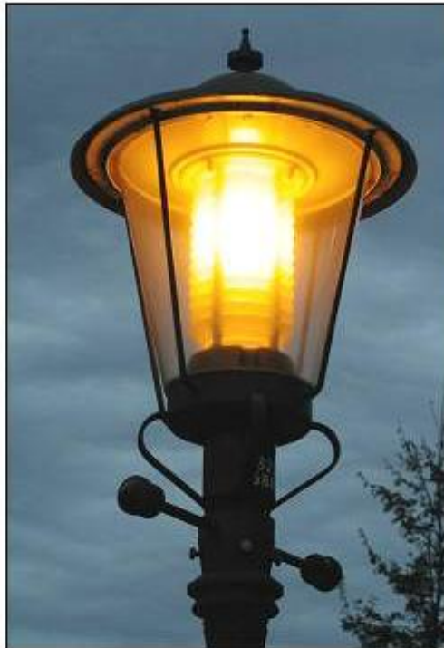
EXISTING LANTERN SON-T 50W
