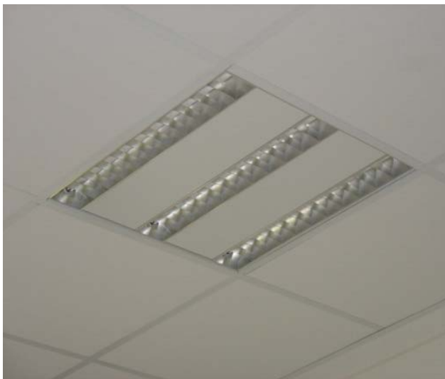
Luminaires with T5 lamps
