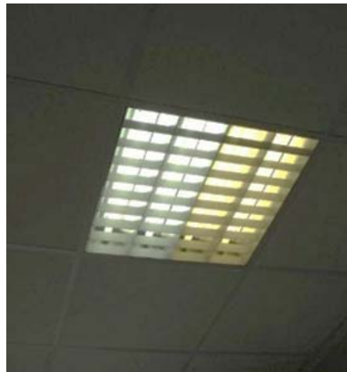
Luminaires with T8 lamps
