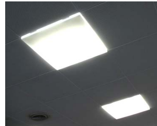
Luminaires with T8 lamps and diffuser
