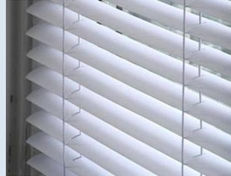
Possibility to adjust the right level of daylight indoor, and, with specific louvre design, to bring daylight deeper into interiors.
