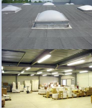
Insufficient daylight, aging roof monitors, steady electrical lighting
