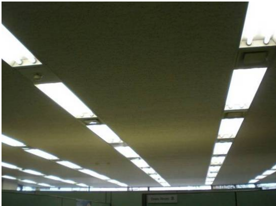
Prior to retrofit 28W/m 2
