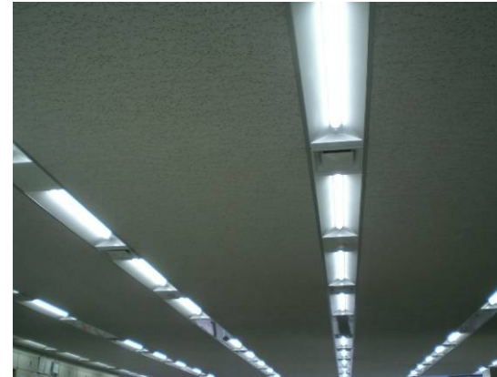
After retrofit 9.6W/m 2 (-66%) (Dimming to setting the right light level )
